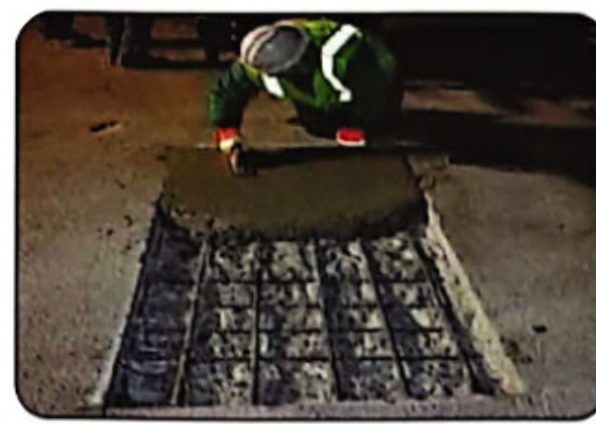
Repair Mortar
