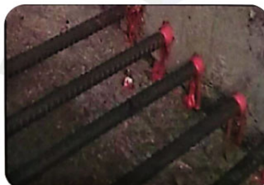
Re-bar Anchoring
