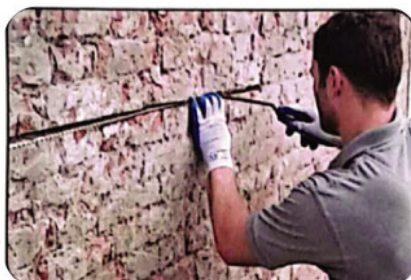
Masonry Wall Repair
