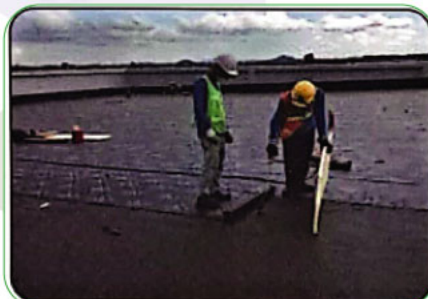
Bituminous Membrane
