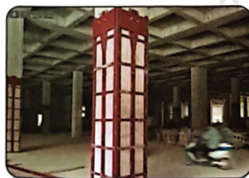
Retrofitting by Steel Plate
