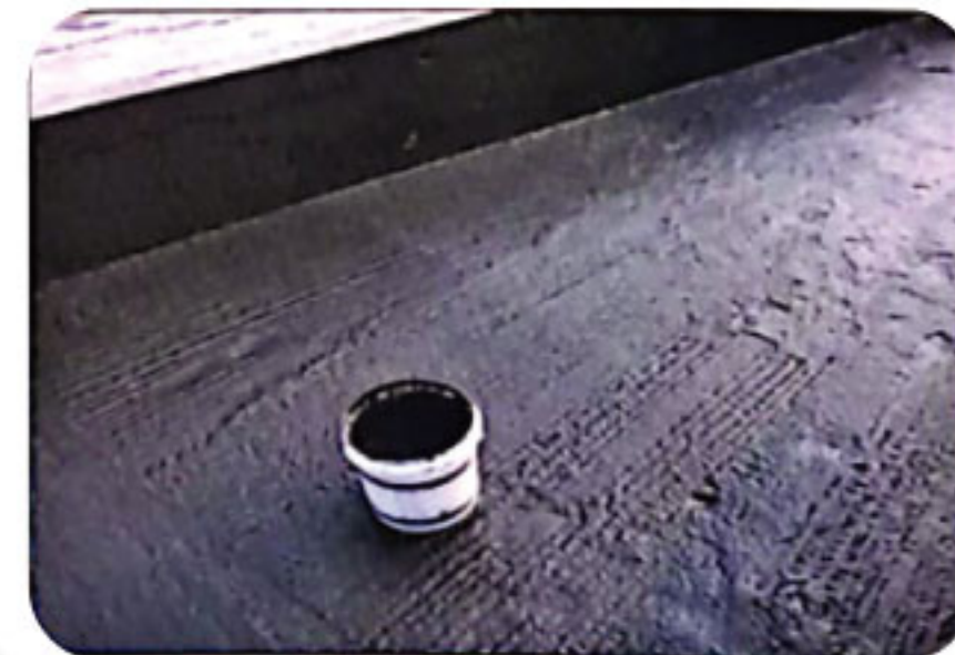
Polyurethane Waterproofing
