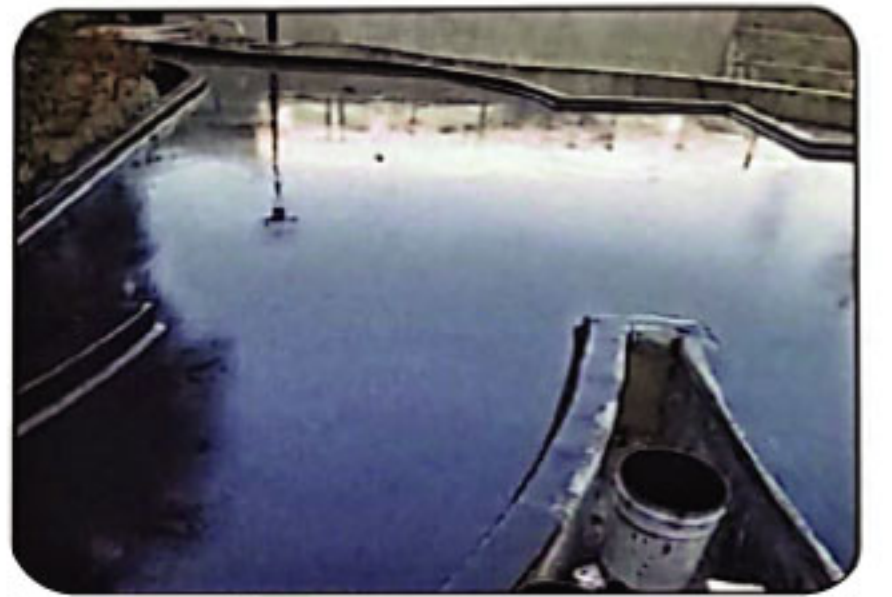
Polyurethane Waterproofing
