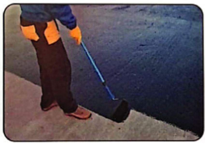
Bituminous Waterproofing
