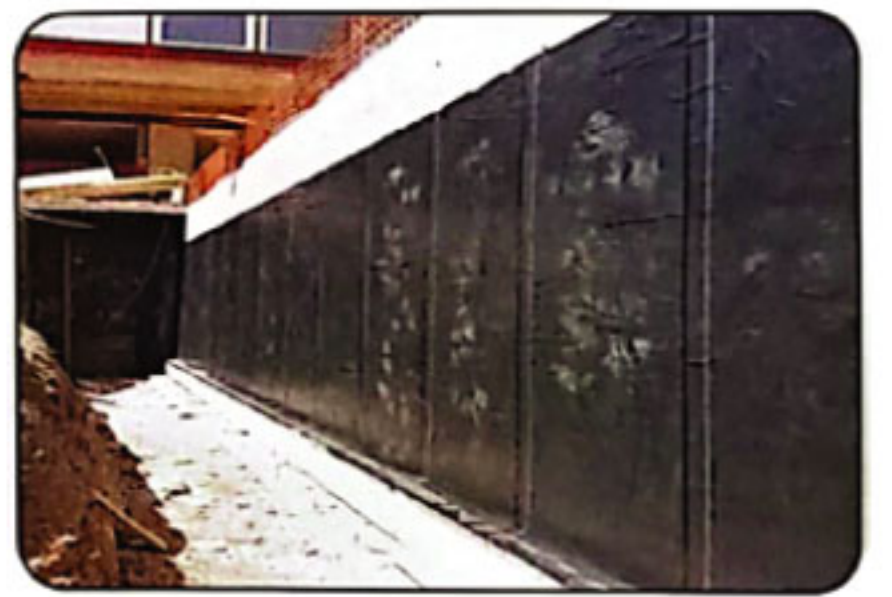
SBS Bituminous Membrane
