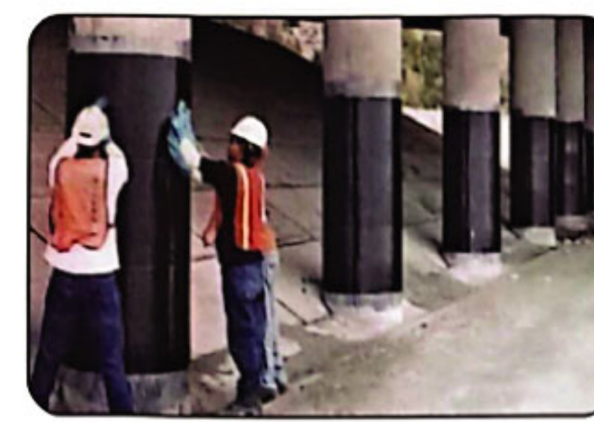
CFRP Retrofitting
