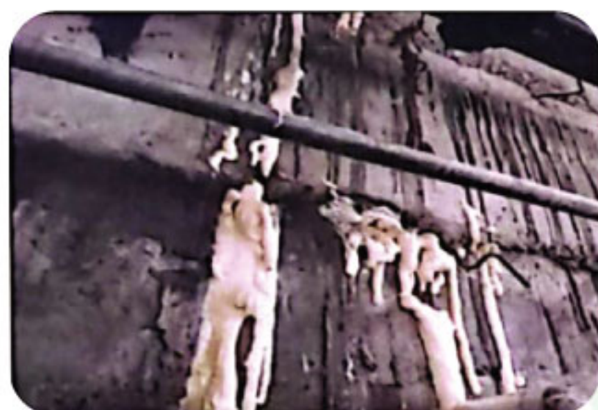
Injection leakage Treatment
