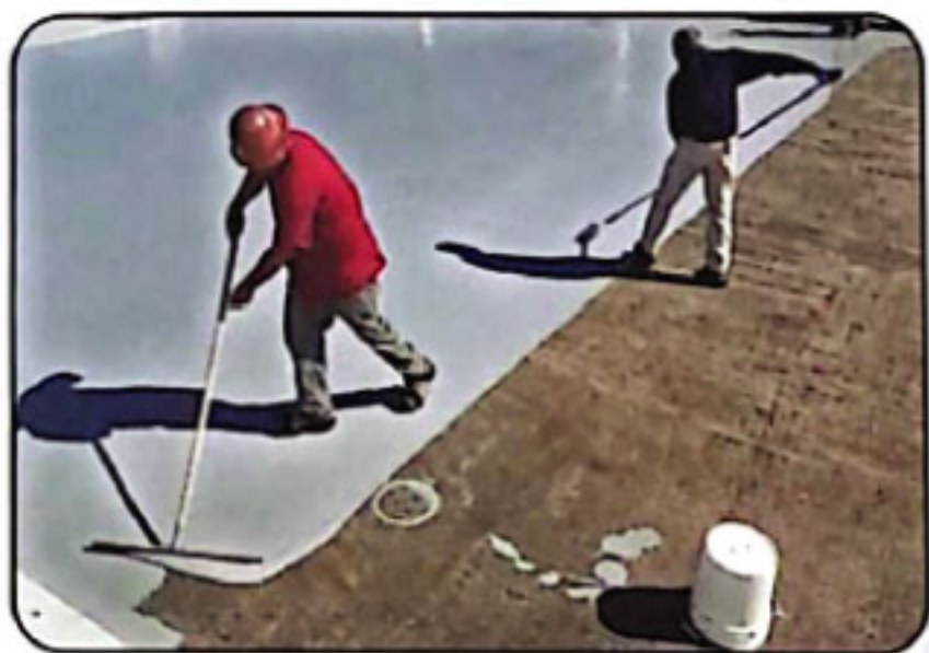
Polyurethane Waterproofing
