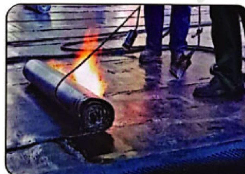
SBS Bituminous Membrane
