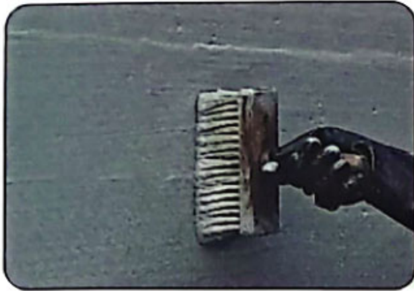
Crystalline Waterproofing
